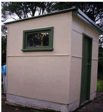
Figure 1: Bonded Asbestos (Fibro)
