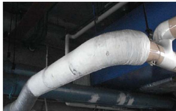
Figure 3: Friable Asbestos – Pipe Lagging
