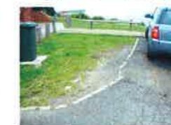
FAILING PAVEMENT
