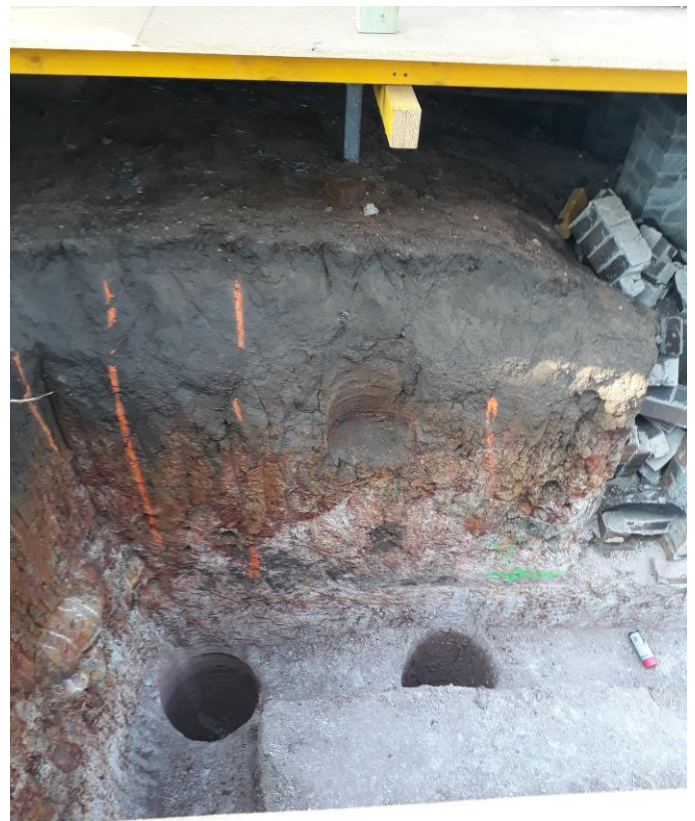
Showing depth of internal pier footings
