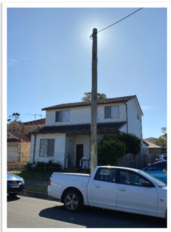
Pole location – 14 George Street
