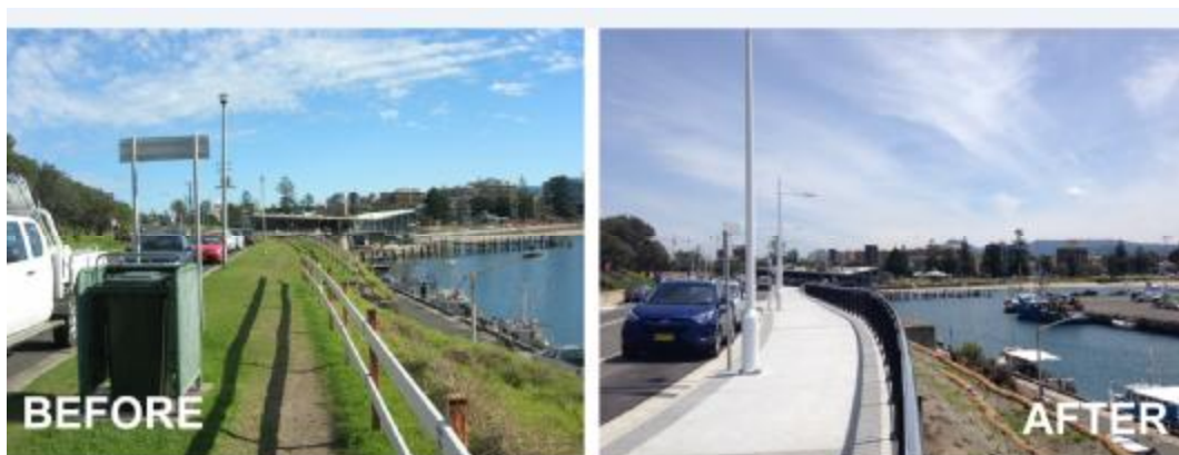
IMAGE: Completed footpath construction at Endeavour Drive, Wollongong
