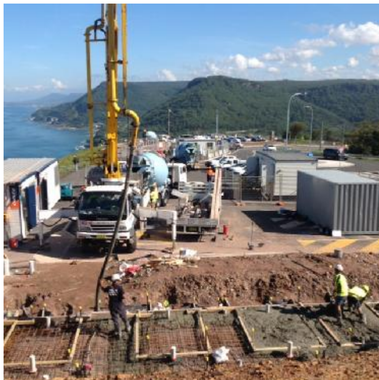
IMAGE: Works progress at Bald Hill Stanwell Park.
