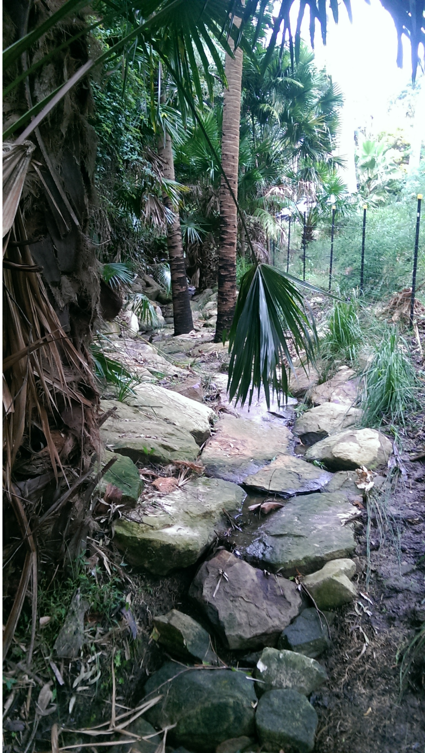
Figure 3: An example of boulders across the channel of a small watercourse as a method of bed erosion protection (Southern Habitat, Newcombe Street, Maianbar, 2015). In the example pictured here, a long stretch of the channel has been engineered, whereas for the purposes of this VRP, only one row of boulders across the channel is needed.
