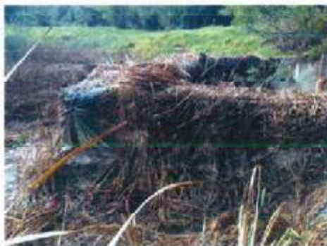
Image 3 Hay bales placed around outlet
