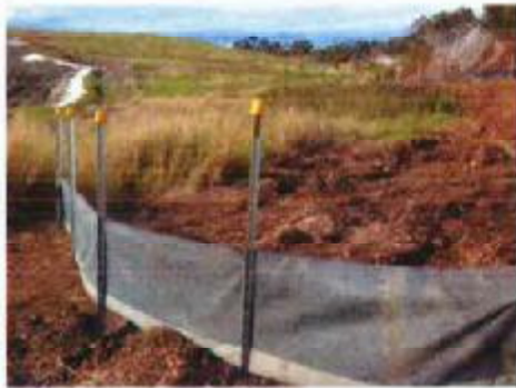
Image 2 Extra sediment fence installation
