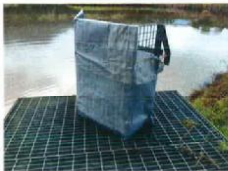
Image 4 Outlet trash basket wrapped in geofabric
