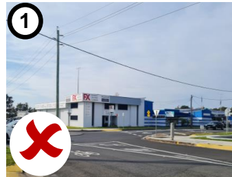
1 Auburn / Swan Street, Wollongong
