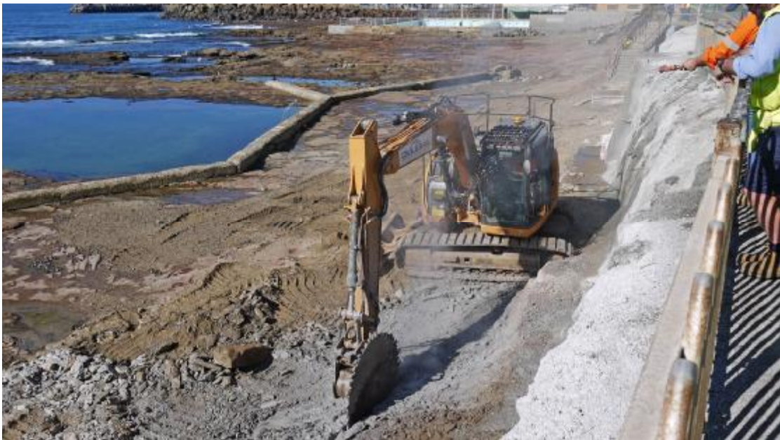
IMAGE: Blue Mile Tramway trenching
