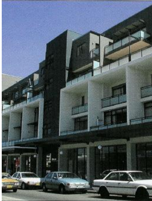
Figure 1: Provides a continuous facade along main commercial streets at the lower levels (Ref: Residential Flat Design Code
