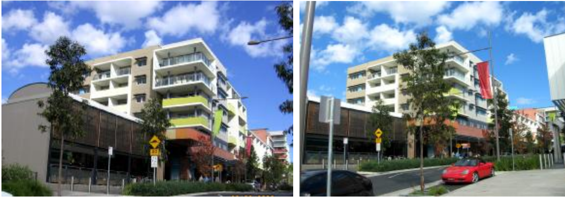
Figures 3 & 4: Mixed use development containing ground floor retail shops and upper residential apartments
