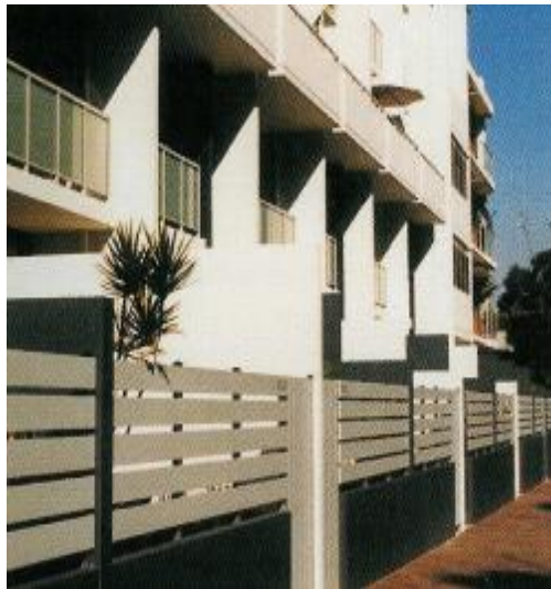
Figure 2: Ground floor residential units with residential entrances directly accessed from the street (Ref: Residential Flat Design Code)
