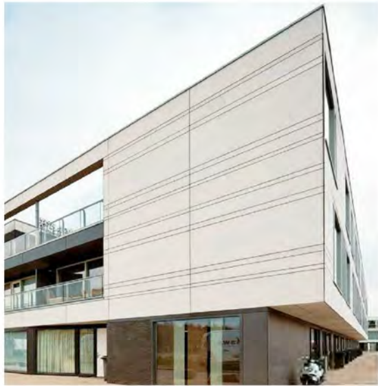
light grey fibre cement cladding (similar to "Cemintel barestone" external pre-finished flat sheet wall cladding)
