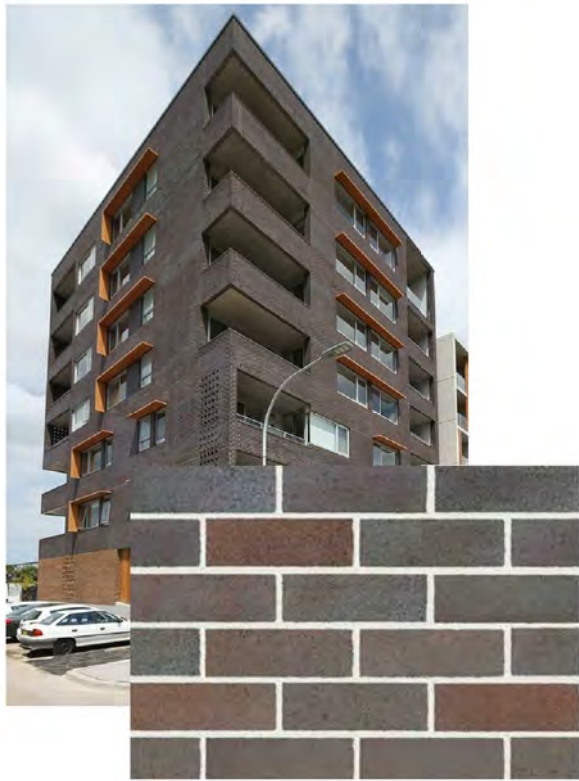
"Bowral Blue" brick facade with light mortar (traditional brick type for heritage precinct)
