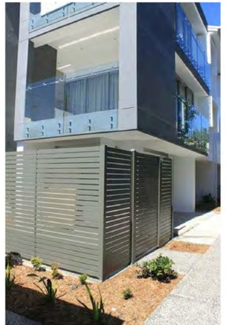
powdercoat "Monument" aluminium slatted privacy screen to ground floor private open spaces
