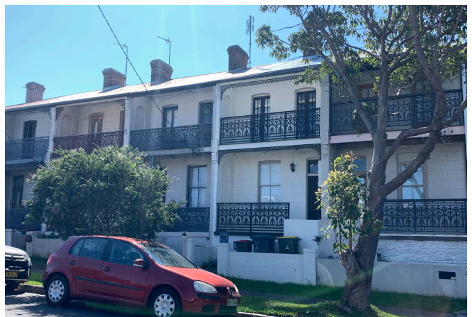
Row of Terraces in Campbell Street, Wollongong
