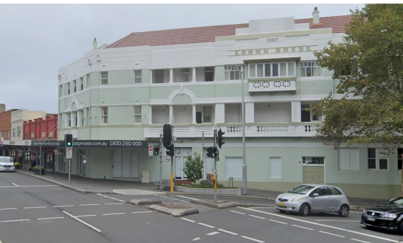
Figure 15: Former Crown Hotel
