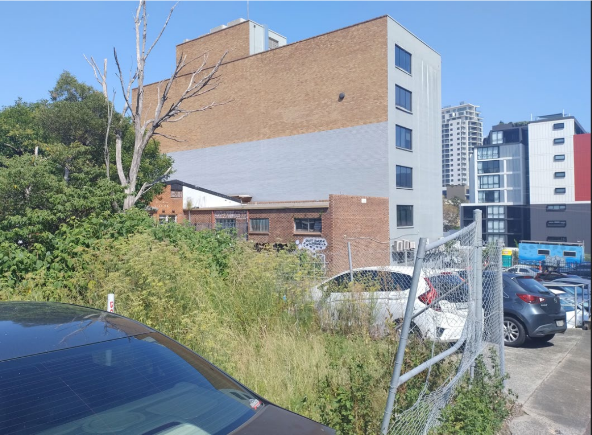
Figure 6: Looking southwest across site from Waters Place
