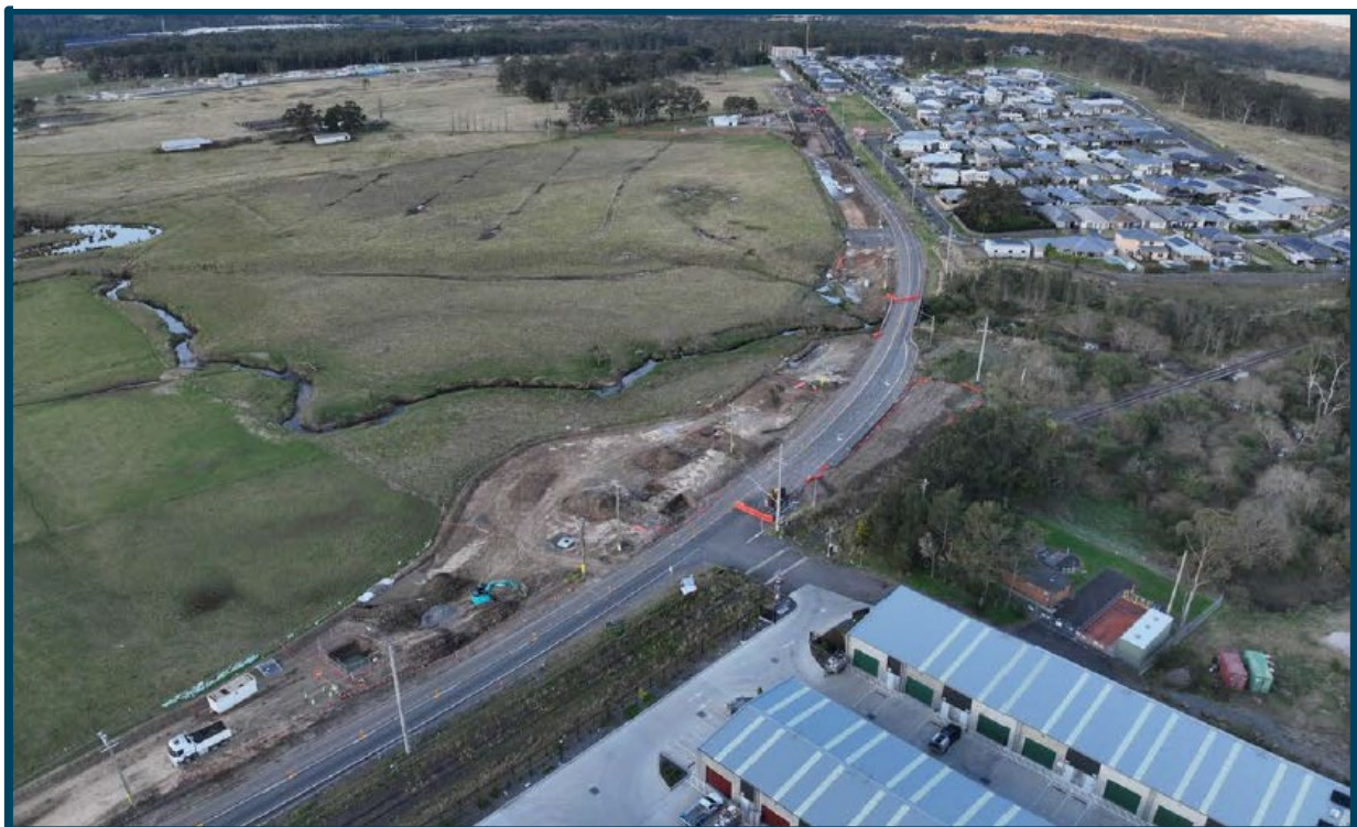
Stage 2 of the West Dapto Road upgrade is underway, improving the Shone Avenue intersection and delivering new road, bridge and drainage works.
