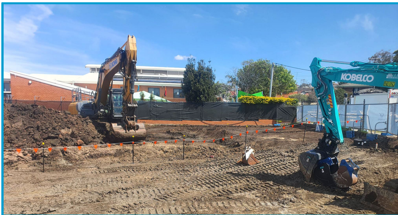
Construction commenced on the landmark Southern Suburbs Community Centre and Library, Warrawong.
