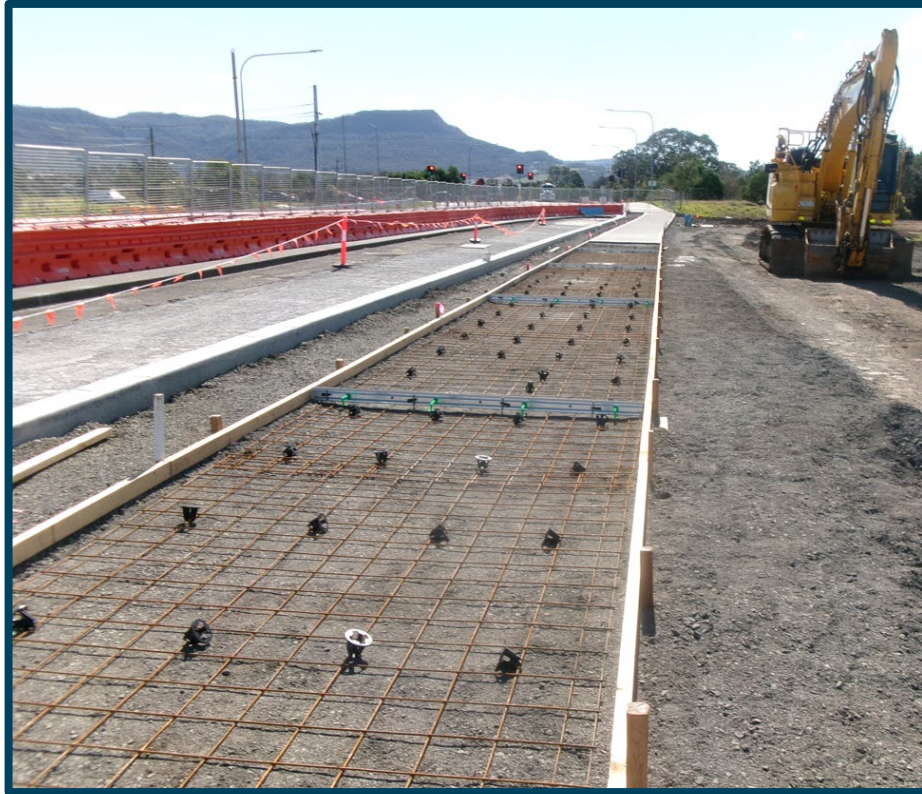
Stage 1 of the Cleveland Road upgrade, West Dapto, is underway, widening 440 metres of road and delivering new and improved shared paths on both sides.
