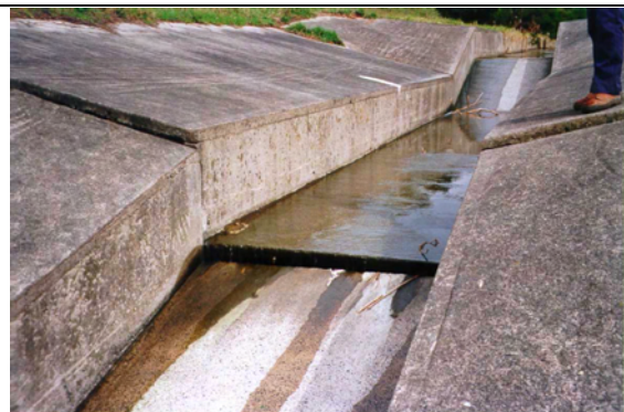
Example of a Steep Concrete Lined Channel
