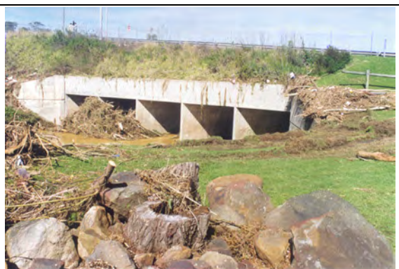
Action for Implementation - Amplification of The Avenue Culverts from existing configuration (shown above)
