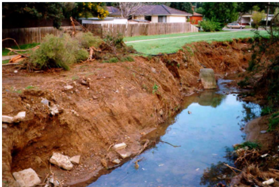
Bank Erosion and Loss of Stabilising Vegetation as a result of August 1998 Flood Event
