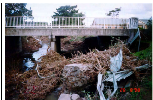
Bank Collapse and Associated Culvert Blockage, Byarong Creek Crossing of Princes Highway, August 1998 Event (Source: Wollongong City Council)
