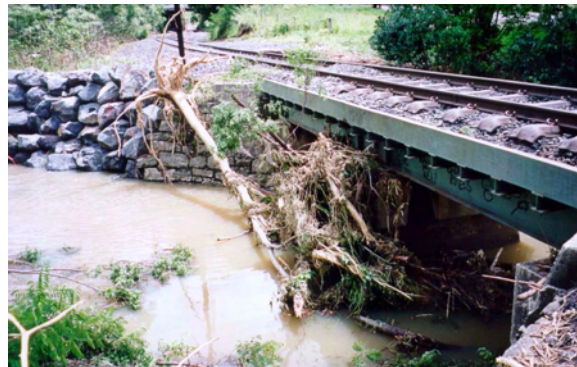
Debris Blocking the Coal and Co Railway Bridge in Upper American Creek
