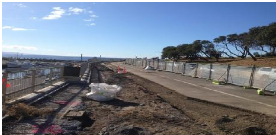
IMAGE: Construction underway for Wollongong Harbour Heritage Walk
