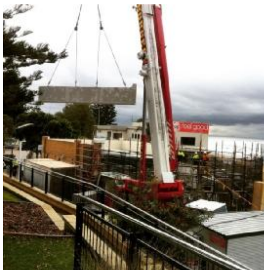
IMAGE: North Beach Kiosk Refurbishment
