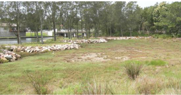
Stormwater quality wetland and detention works integrated along the riparian zone incorporating native re-vegetation and passive recreation and community involvement through ongoing bush regeneration of the wetland
