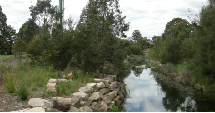
Stream health improvement works including bank restoration and re-vegetation. The image shows combination of hard and soft elements to prevent ongoing erosion in areas of steep banks and active erosion.
