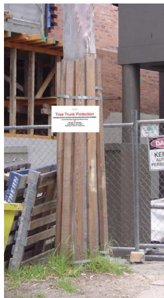
Plate 5: Example of trunk protection with sign attached, recommended for Tree 1. P. Vezgoff.
