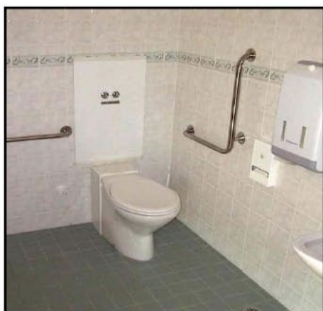
Figure 30: The incorrect placement of the toilet paper holder too far forward of the WC pan, which forces patrons to lean excessively forward to get to the paper. This can result in patrons falling off the pan in attempting to reach the toilet holder.
