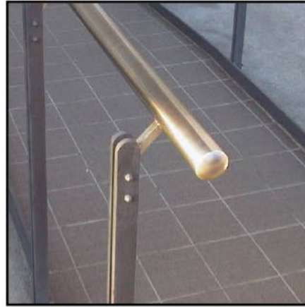
Figure 5: (Top left) Handrails which do not comply with the specifications of AS1428.1 for handrails on stairs suitable for people with disability since the handrails fail to return to a side wall or downwards and back on themselves at 180°.
