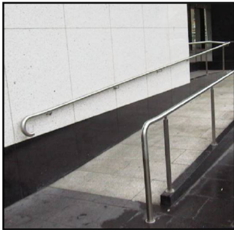
Figure 3: (Top left) Correct application of returning the handrail down and back onto itself to form 180° return onto a post. The handrails also provide clearances on the top 270° arc of the handrail and the 15mm directly under the handrail to allow for uninterrupted transition along the full length of the handrail for fingers and thumbs.
