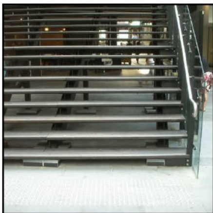
Figure 11: (Top left) Open risers and light sources coming from behind the stairway impact upon contrast and present a space for mobility aids to become unintentionally lodged.
