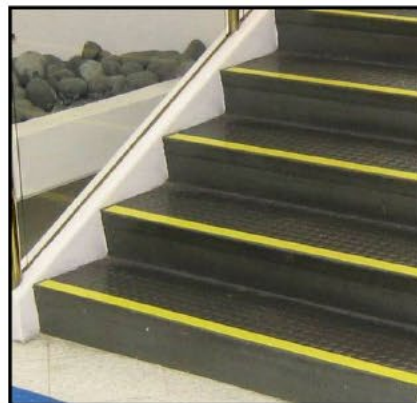
Figure 9: (Top left) The correct minimum luminance contrast and depth of treatment on the nosings of the treads / goings.
