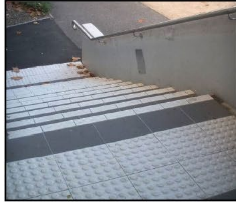
Figure 16: (Top left) TGSIs which have a high luminance contrast, as required by AS 1428.4. The photographs also show the correct setback from the top nosings of 300 +/- 10mm and the minimum depth of 600mm.
