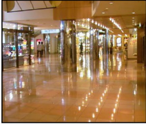
Figure 22: (Top left) Very shiny and slippery floor surfaces which fail to meet the "R" rating, as required by AS4586 and HB197.
