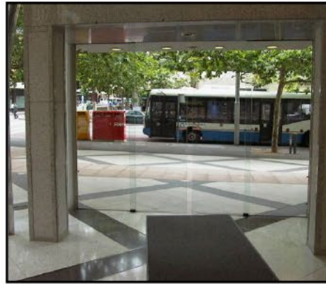
Figure 22: (Top left) Very shiny and slippery floor surfaces which fail to meet the "R" rating, as required by AS4586 and HB197.
