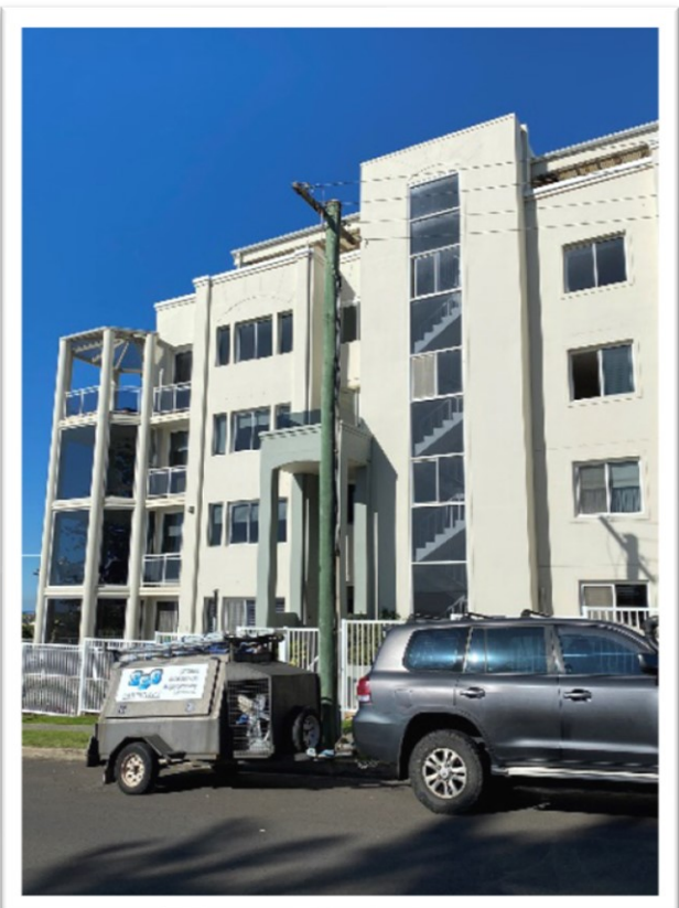
Pole location – Georges Place
