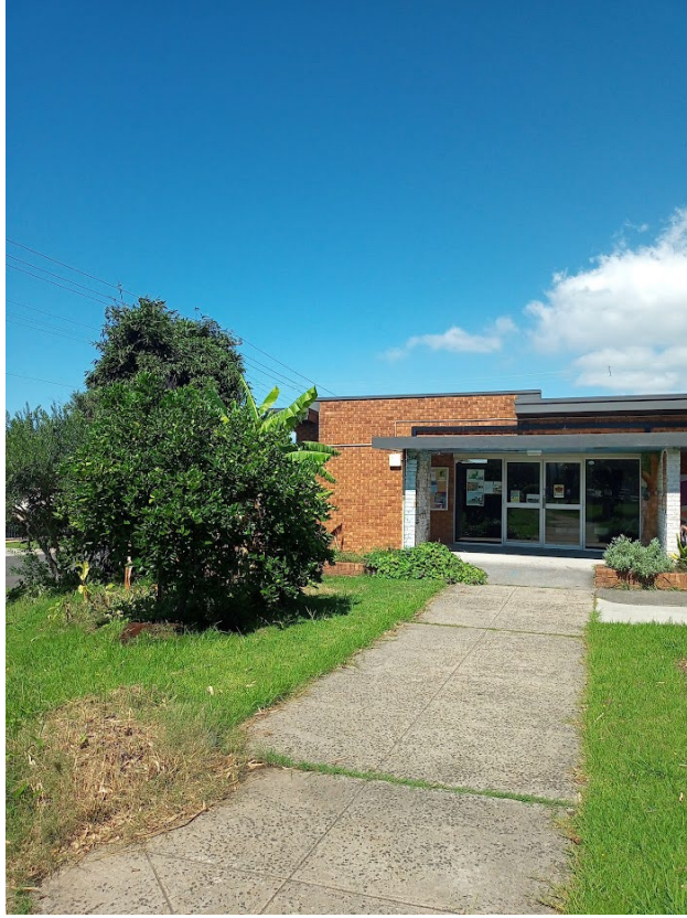
View of existing hall building entrance
