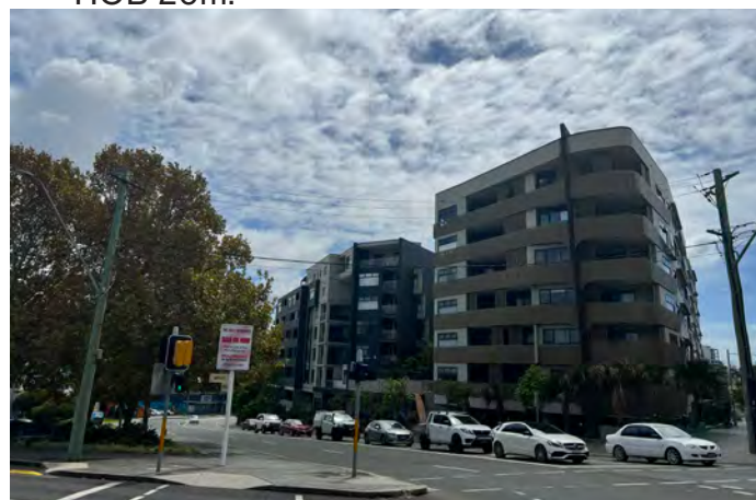
⑨ 83 Campbell Street and 65-73 Flinders Street, Wollongong Completed at the end of 2020, HOB 31m.
