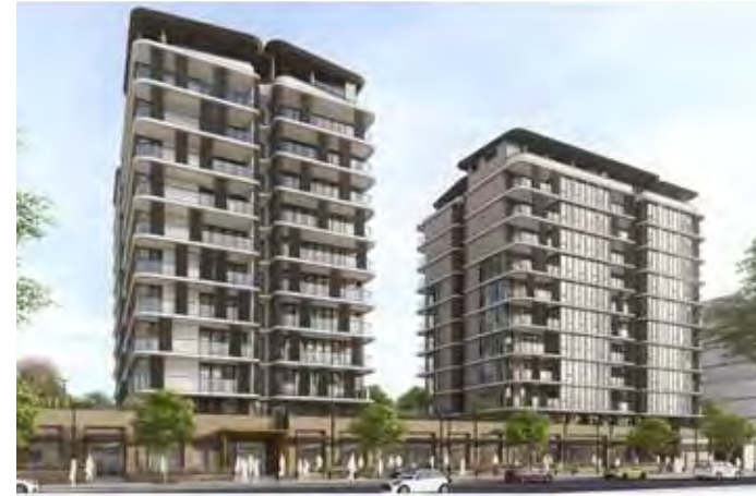
② 36 Flinders Street, Wollongong Currently under construction.
