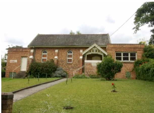
Figure 7.6 The Uniting Church at 48 Moore Street
