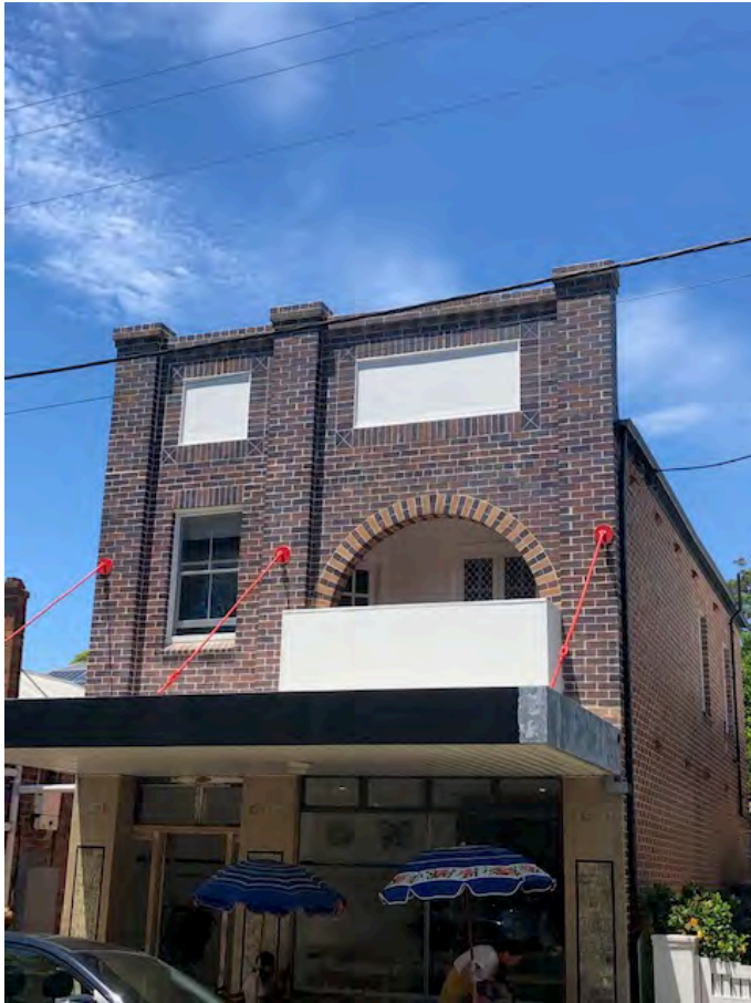
Figure 3: Site Inspection Moore Street frontage
