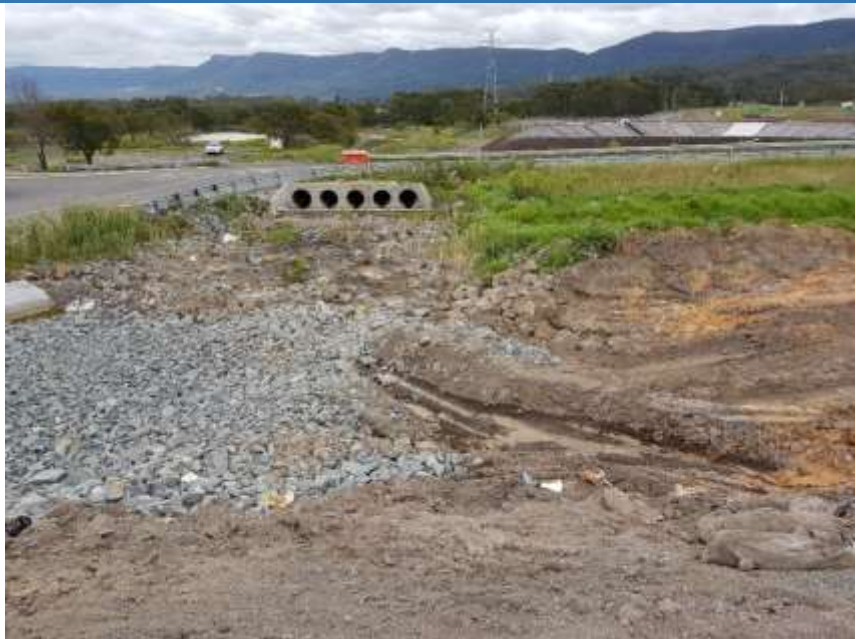
Photo below was taken at the new leachate pond noting the scouring along the toe of the embankment.
