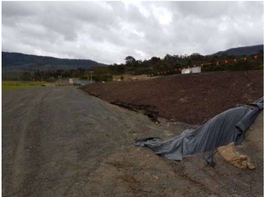
Photo below was taken at the new leachate pond noting the scouring along the toe of the embankment.
