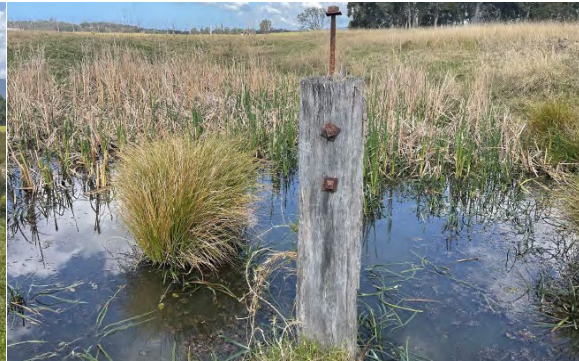
Figure 22 Wooden pier likely associated with the railway bridge.
