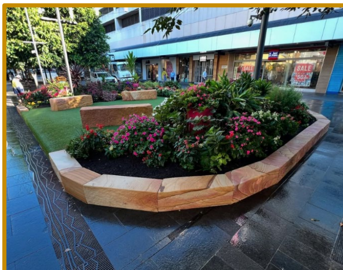
The Crown Street Mall Parklet received a refurbishment with the edging being replaced with flat-topped sandstone blocks.
