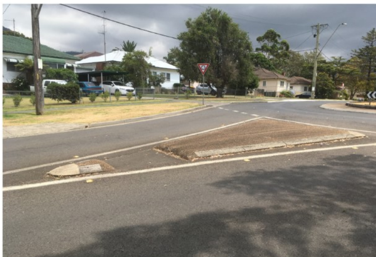
Gap in traffic island is too small to accommodate wheelchairs, prams or bicycles
