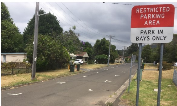
Existing Parking Bay Linemarking
