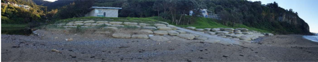
Figure 7 Geotextile Bag Wall at Southern end of Coalcliff Beach
