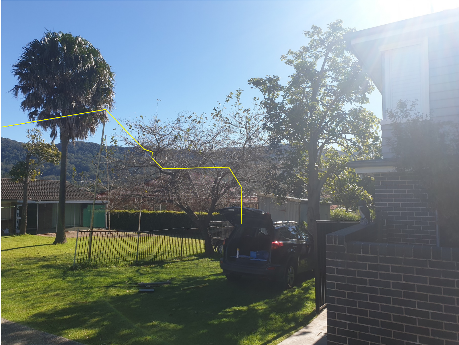
Alternate view from boundary with No.23 Russell Street, with roof line of proposed dual occupancy shown yellow.
