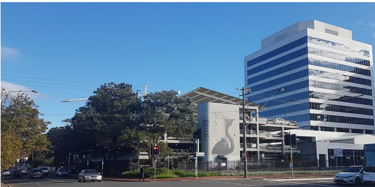
[IMAGE: Council's Administration Car Park Solar Project, Stewart Street Wollongong]
