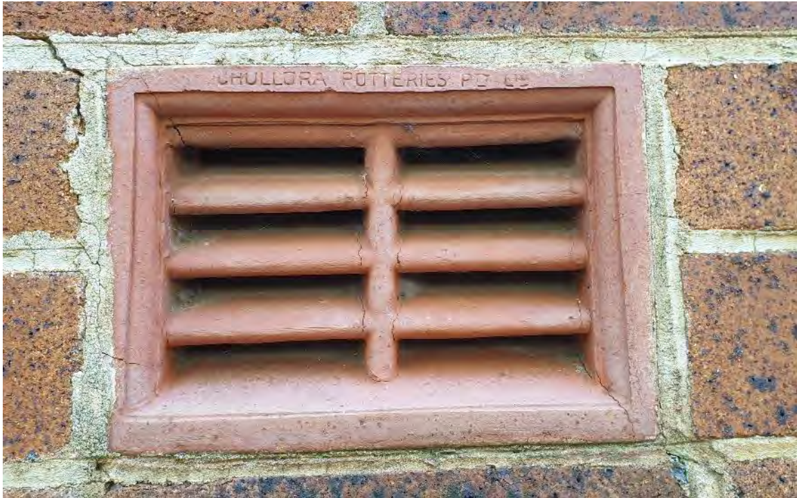
Figure 5.8 Photograph of the Chullora Pottery vents.
