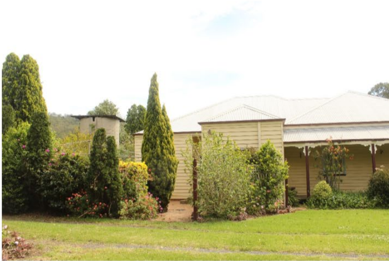
Figure 10: Southern façade showing recent additions to left of image, with the original veranda configuration and hipped roof form (right of image). Note the position of the silo to far left.
