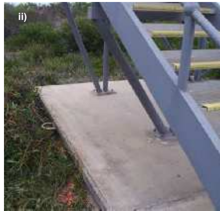
Figure 2. i) Patrol tower at Corrimal Beach ii) Precast footing showing hooks to drag the structure.
