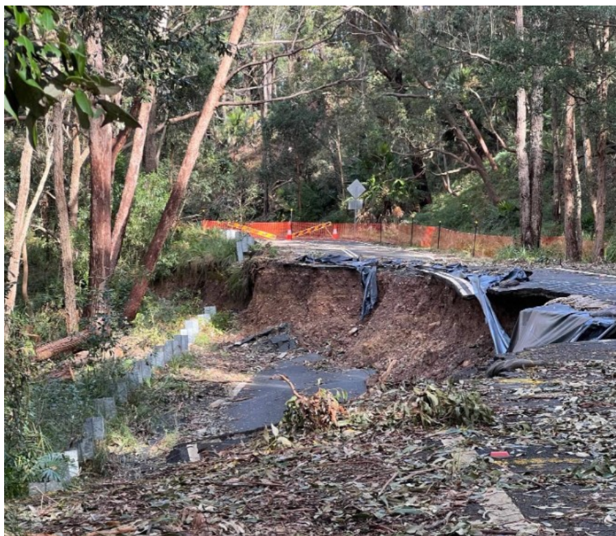
Image: Landslip damage on Garie Road in the Royal National Park
