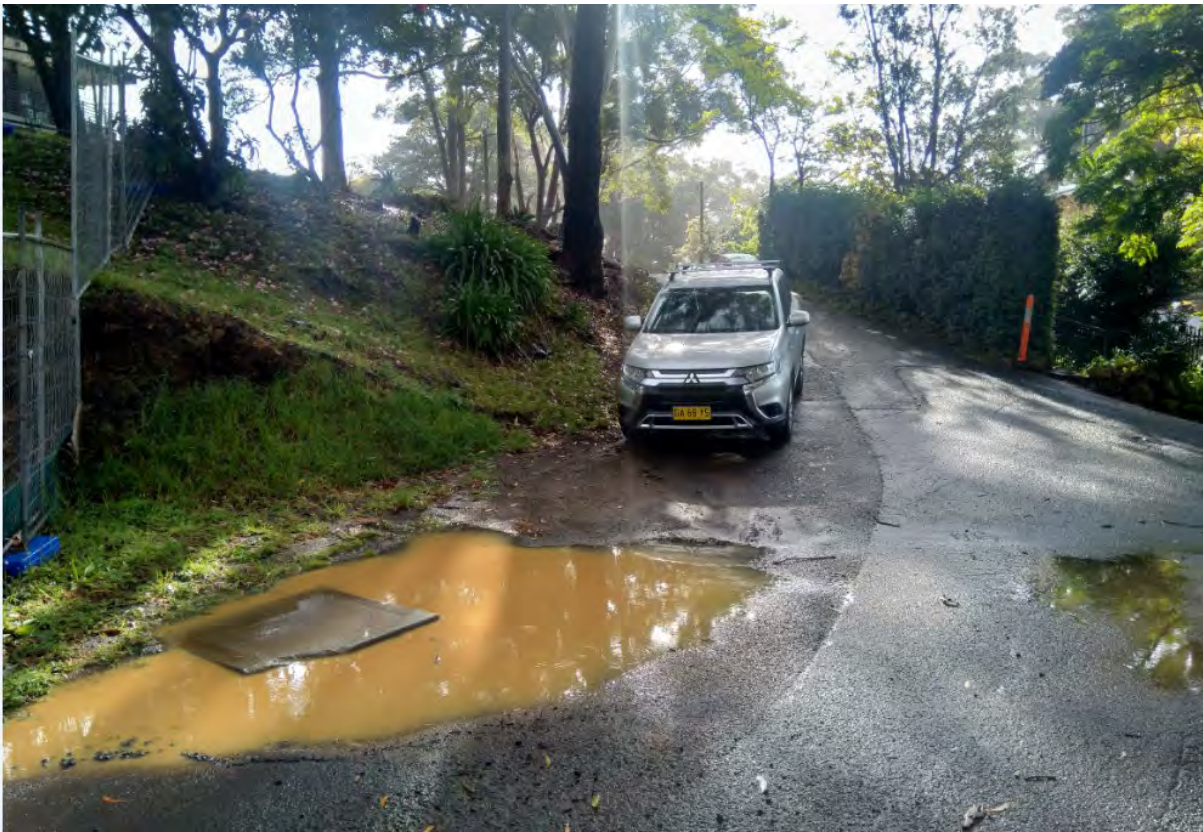
Figure 3: View looking west along Norman Street from subject site
