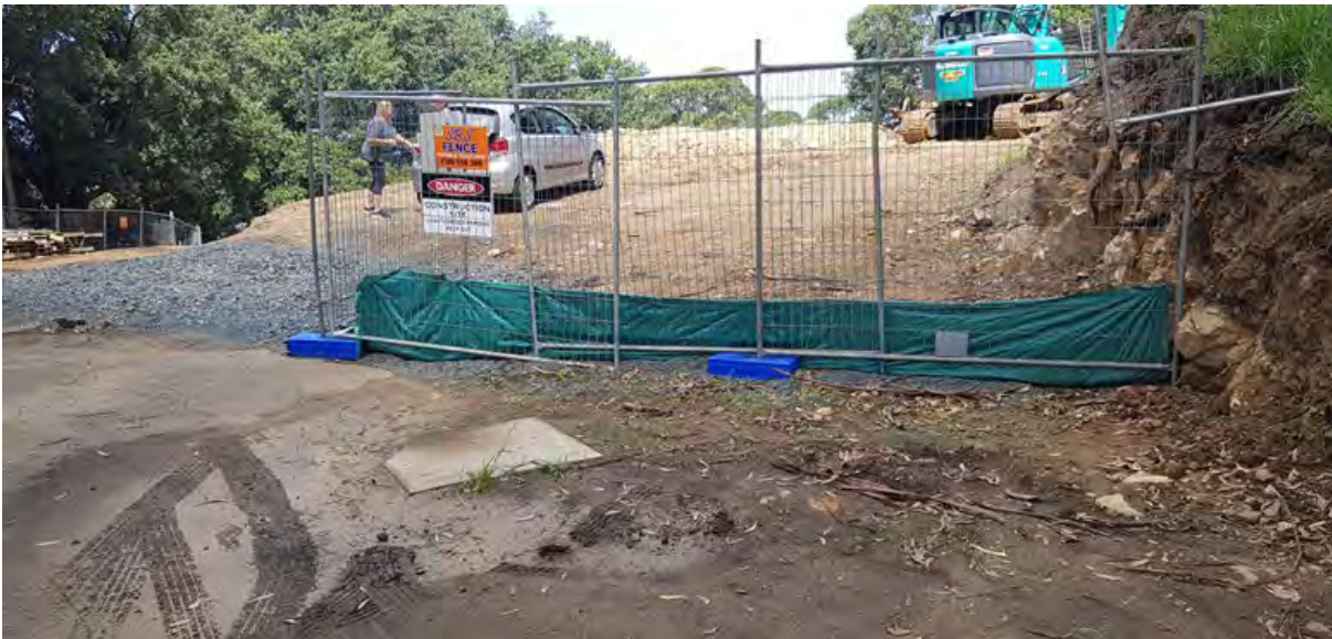
Figure 4: View towards the site from Norman Street with decommissioned stormwater pit in foreground
