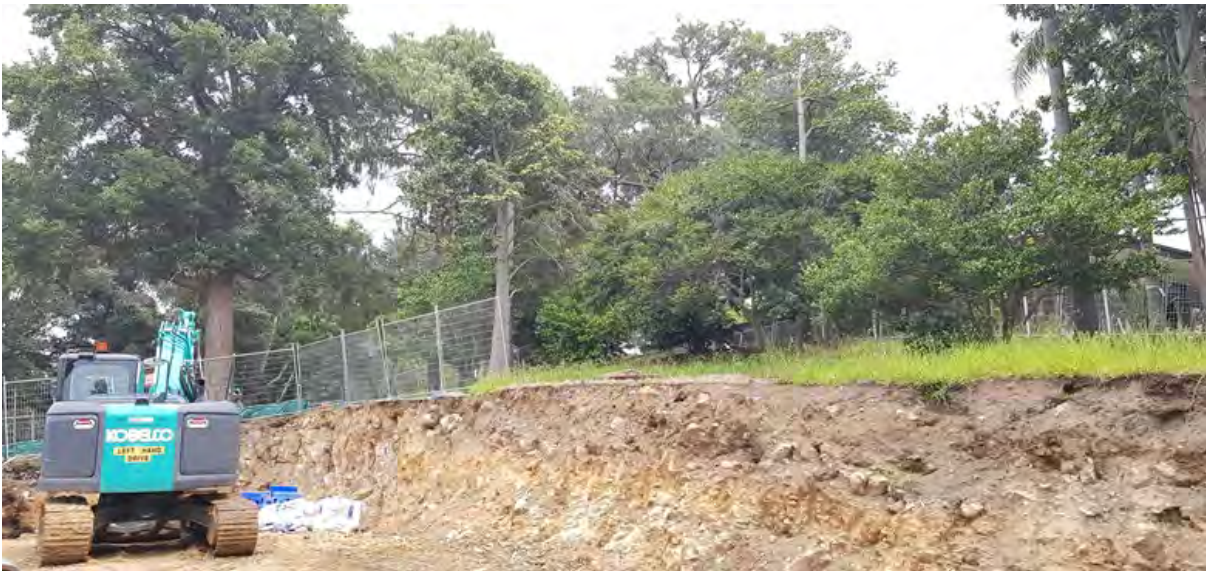
Figure 1: View looking south along western boundary of the site with Turpentine T1? tree to left of shot
