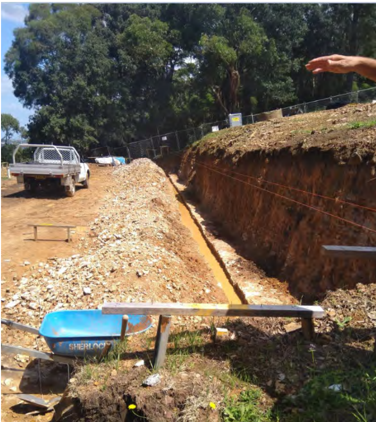
Figure 8: View looking south along excavation for retaining wall towards Council reserve
