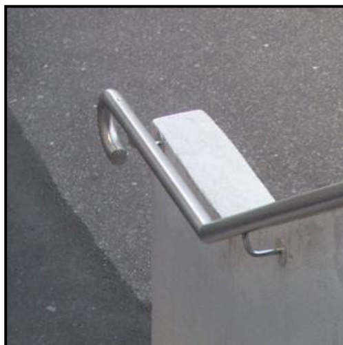
Figure 7: (Top left) Correct return of the handrail to a side wall and the required 270° top arc clearance.
