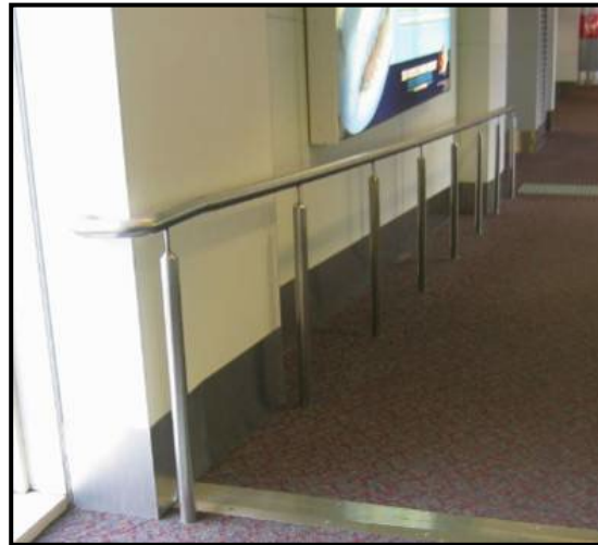
Figure 3: (Top left) Correct application of returning the handrail down and back onto itself to form 180° return onto a post. The handrails also provide clearances on the top 270° arc of the handrail and the 15mm directly under the handrail to allow for uninterrupted transition along the full length of the handrail for fingers and thumbs.
