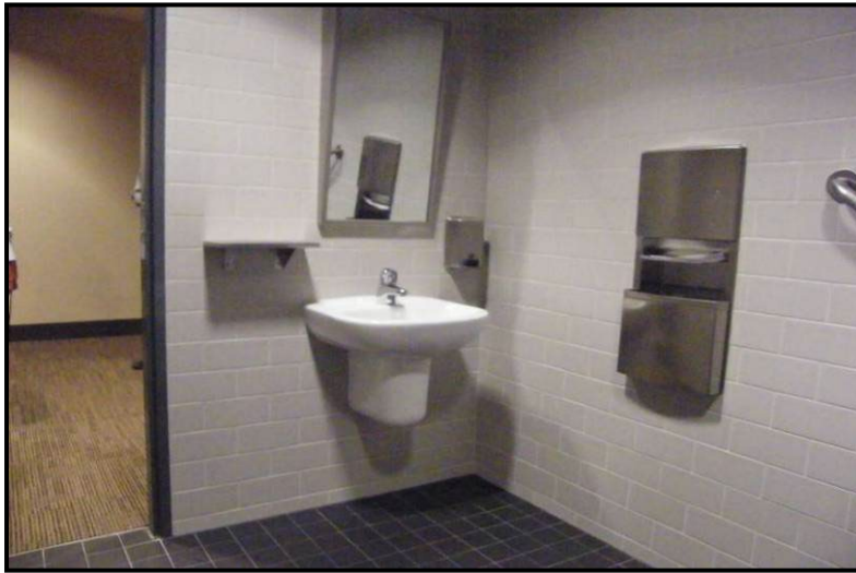
Figure 29: The correct installation of a washbasin and other fittings, including a shelf as required by Table F2.4 of the BCA.
