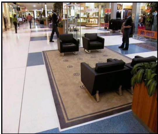
Figure 24: (Top left) Show floor surfaces which meet the “R” rating under AS4586 and HB197.
