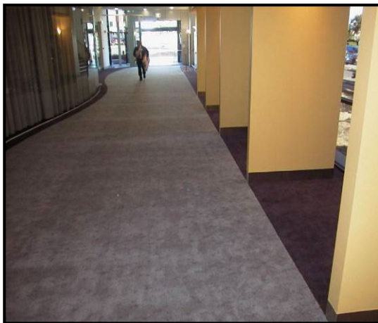
Figure 24: (Top left) Show floor surfaces which meet the “R” rating under AS4586 and HB197.
