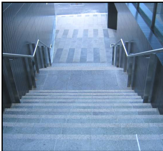
Figure 18: The correct interpretation of the requirements for TGSIs on an intermediate landing with no handrail break: there are no TGSIs on the landing.
