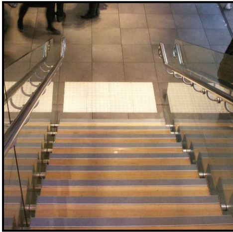
Figure 9: (Top left) The correct minimum luminance contrast and depth of treatment on the nosings of the treads / goings.
