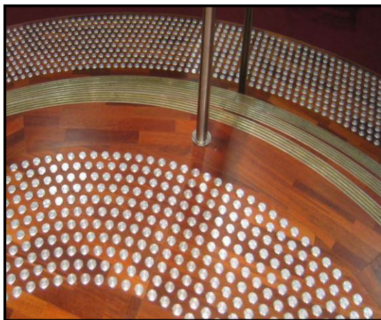
Figure 16: (Top left) TGSIs which have a high luminance contrast, as required by AS 1428.4. The photographs also show the correct setback from the top nosings of 300 +/- 10mm and the minimum depth of 600mm.
