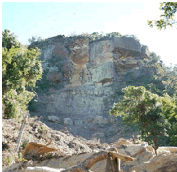
Rockfall below Five Islands Lookout showing overhanging area of the cliff. Source: Phil Flentje, University of Wollongong
