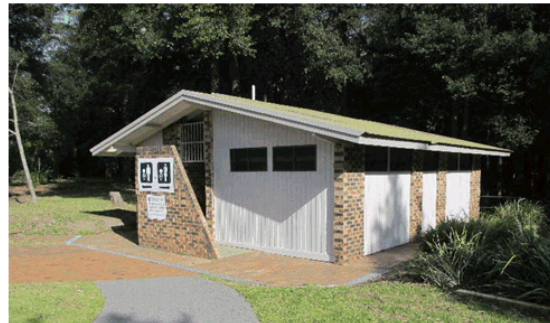
Toilet block at Mt Keira
