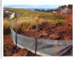
Image 2 Extra sediment fence installation
