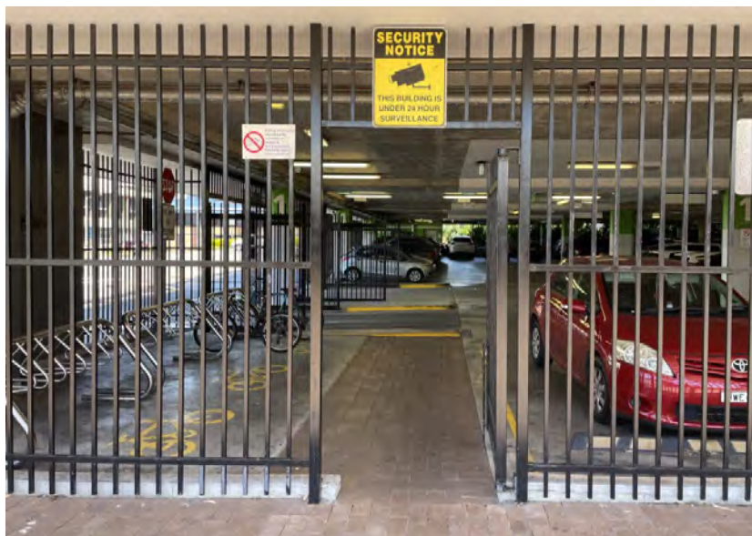
Figure 75: Bicycle parking facilities should have a safe path of travel to entry/ exit points.
