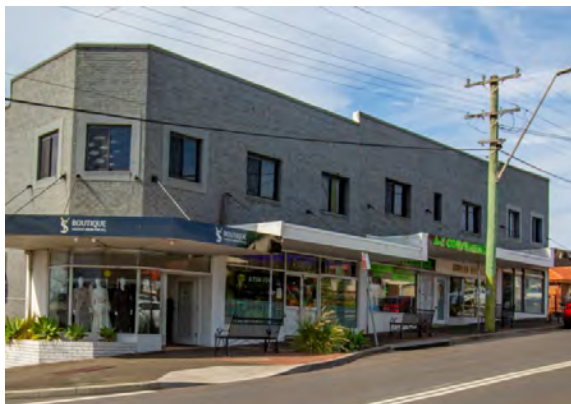
Figure 51: Awnings along a sloped site should step down with the topography, while providing continuous weather protection for pedestrians.
